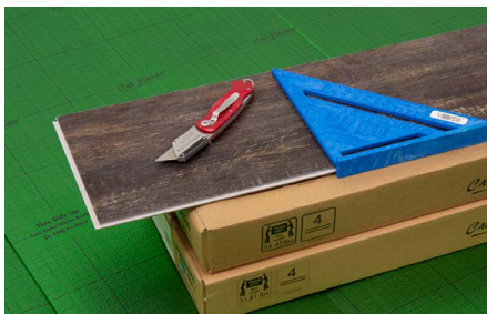
Cutting boards using Score and Snap technique
