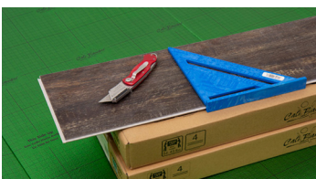
Cutting boards using Score and Snap technique
